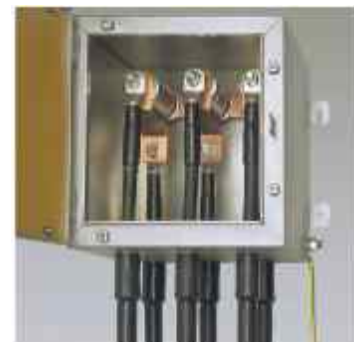
Link box installed with cross bonding cables
